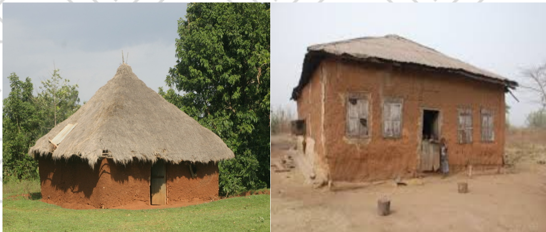
Figure 2.2: A Traditional Hut in Africa Built with Laterite Soil and Thatch Roof. (Google, June 2012)
